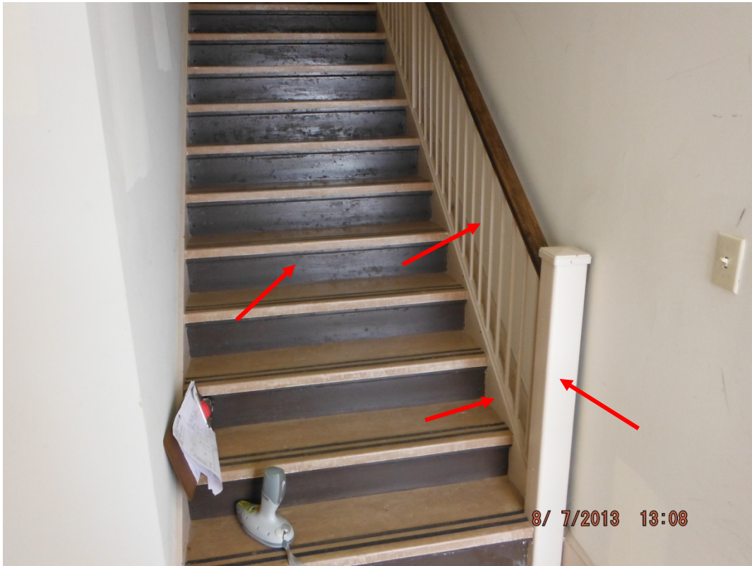
Stair newel post, balusters, risers, and stringers
