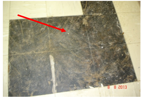
Photo 2. Asbestos-containing black mastic under non-ACM 12"x12" floor tiles was found in various areas of the subject structure. An area of exposed black mastic was observed in the basement mechanical room (002) as depicted herein.
